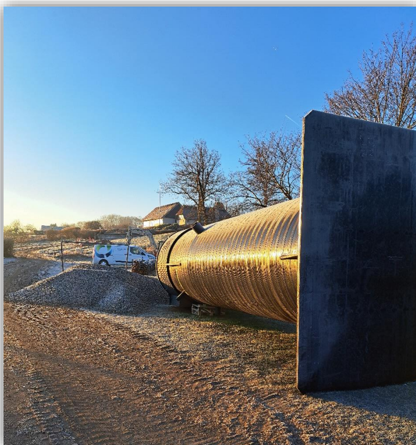
Ny pumpestation Mørkholt - Hagenvej
